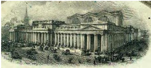
Pennsylvania Station, New York City
