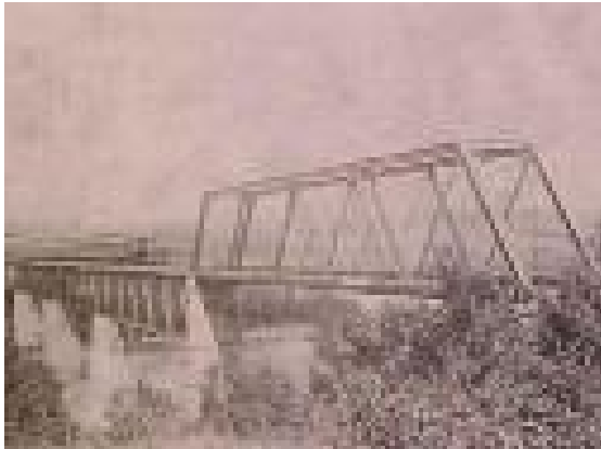
Railroad Bridge in Loudon, Tennessee.
